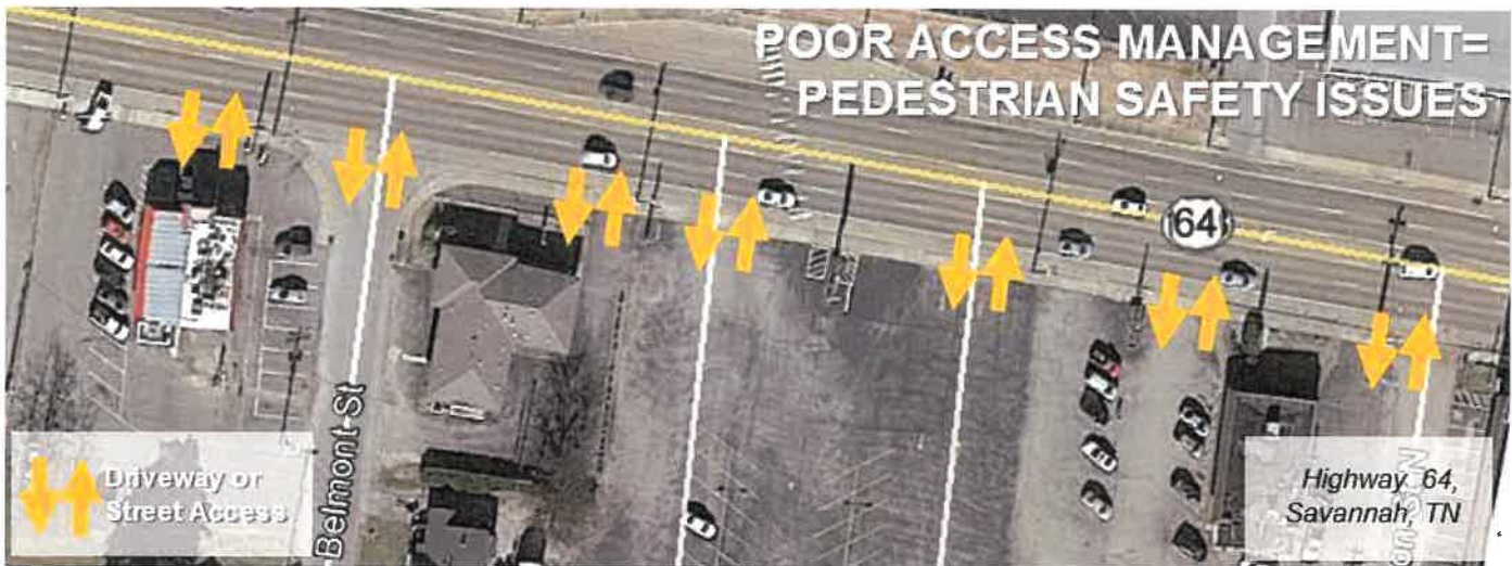
Figure 38 Example of Poor Access Management
