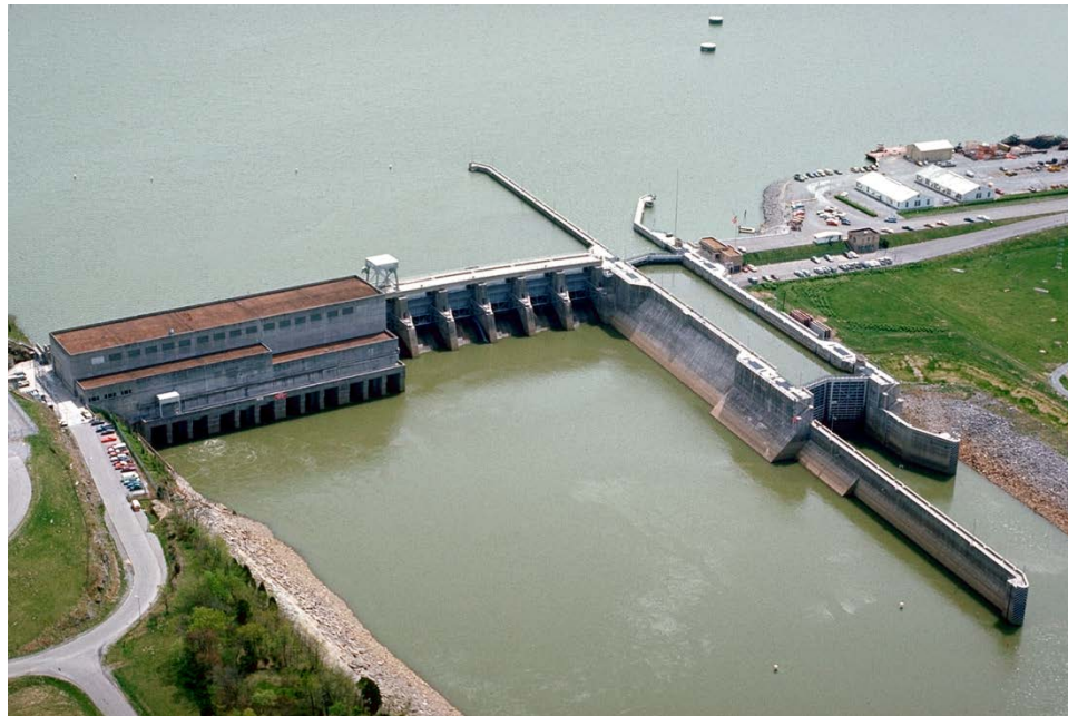
Figure 3- Old Hickory Lock and Dam
