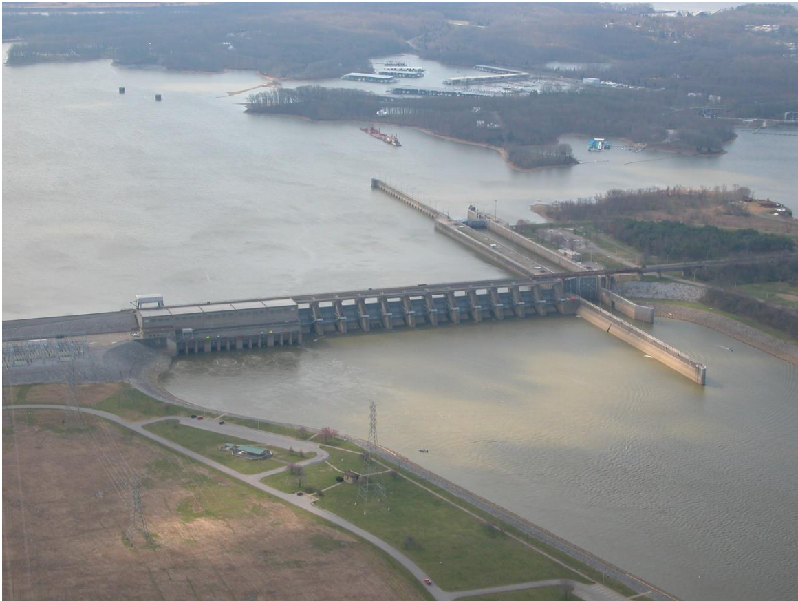
Figure 1.1 - Barkley Lock and Dam Project
