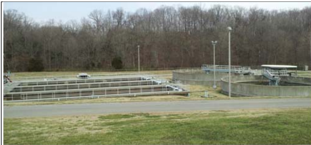
Jones Creek Wastewater Treatment Plant
