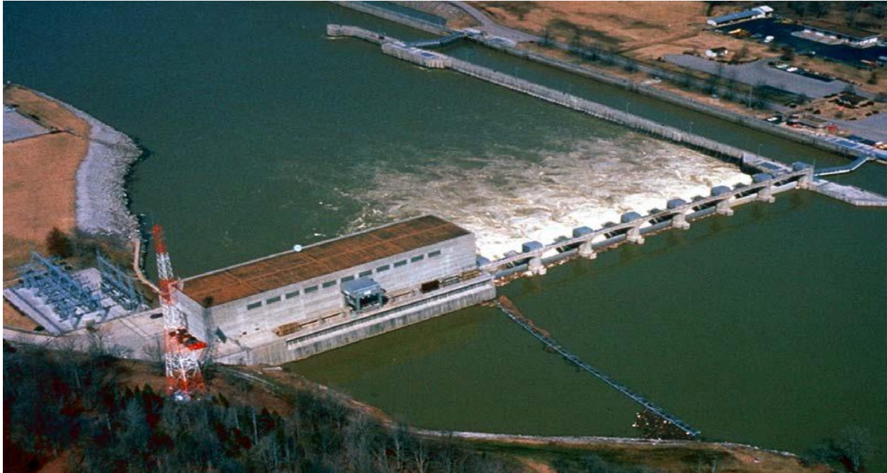
Figure 1.1 - Cheatham Lock and Dam Project
