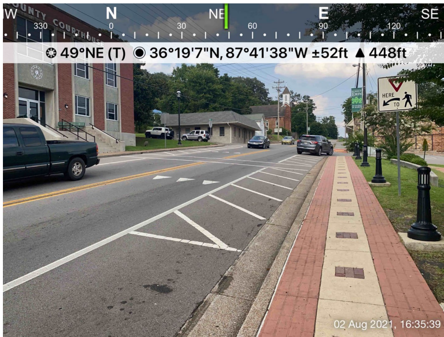
Figure: Existing transverse crosswalk, no-parking area, and pedestrian yield sign.
